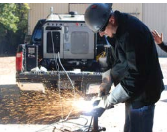
Handheld cutting in the field
